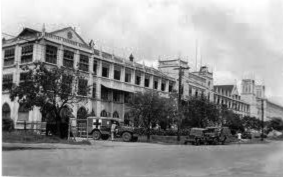
Figure 7: Influenza. University of the Philippines pre WW II, where Wade and Manalang conducted their landmark study
